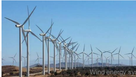
Wind energy system
